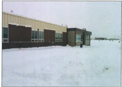
Supervision and lighting level is an issue on the North side of the modular classrooms.
