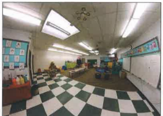
The school has a large central core of instructional spaces with no natural lighting or ventilation.
