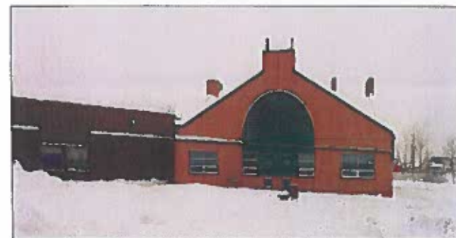
Pooling occurs on the site at the South modulares during spring thaw. Lighting levels should also be improved in this area.
