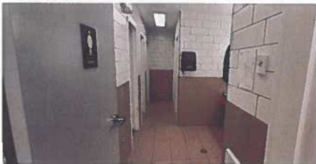
Staff washrooms have been expanded.
