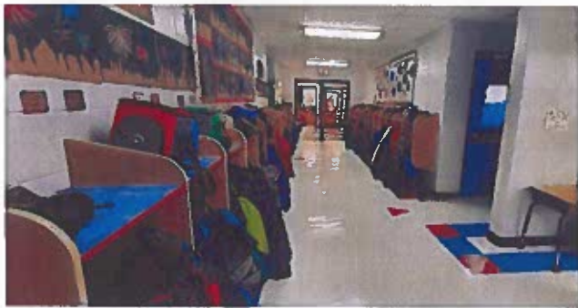
There is a lack of corridor space for cubbies and hooks.
