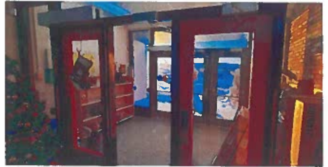
The main entrance of the school suffers from a lack of crush space that causes congestion for students, parents, and visitors.
